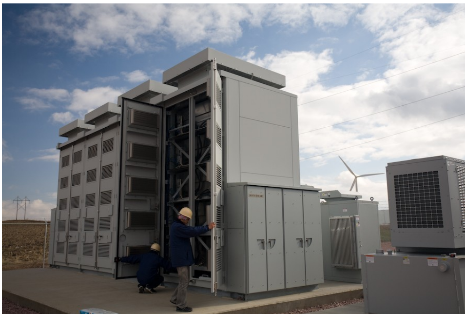
Another view to give a sense of scale. The PCS can be seen behind the battery. The backup generator is on the near right. One of the turbines powering the battery can be seen in the distance.
